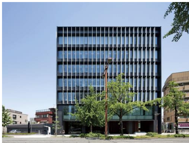
Panoramic view of the Headquarters building ( Features an energy-saving design )
